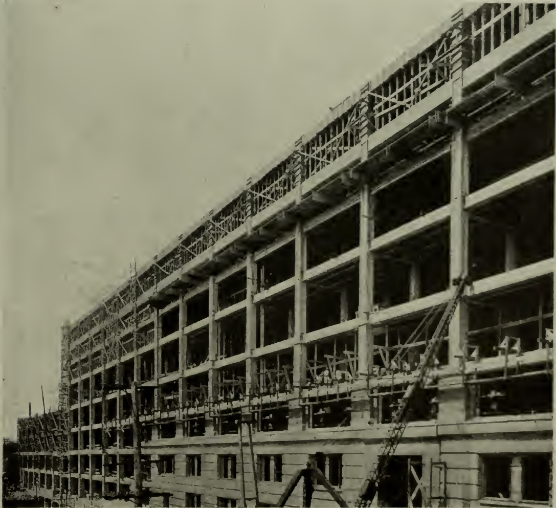
REINFORCED CONCRETE BOTTLING BUILDING, ST. LOUIS: DURING CONSTRUCTION. (See p. 781.)
